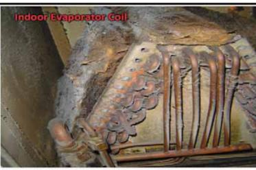
The above picture is a indoor coil; it's part of your air conditioning system. It's hidden in your air duct system so you cant see it ... out of site out of mind. The air you breath is going
